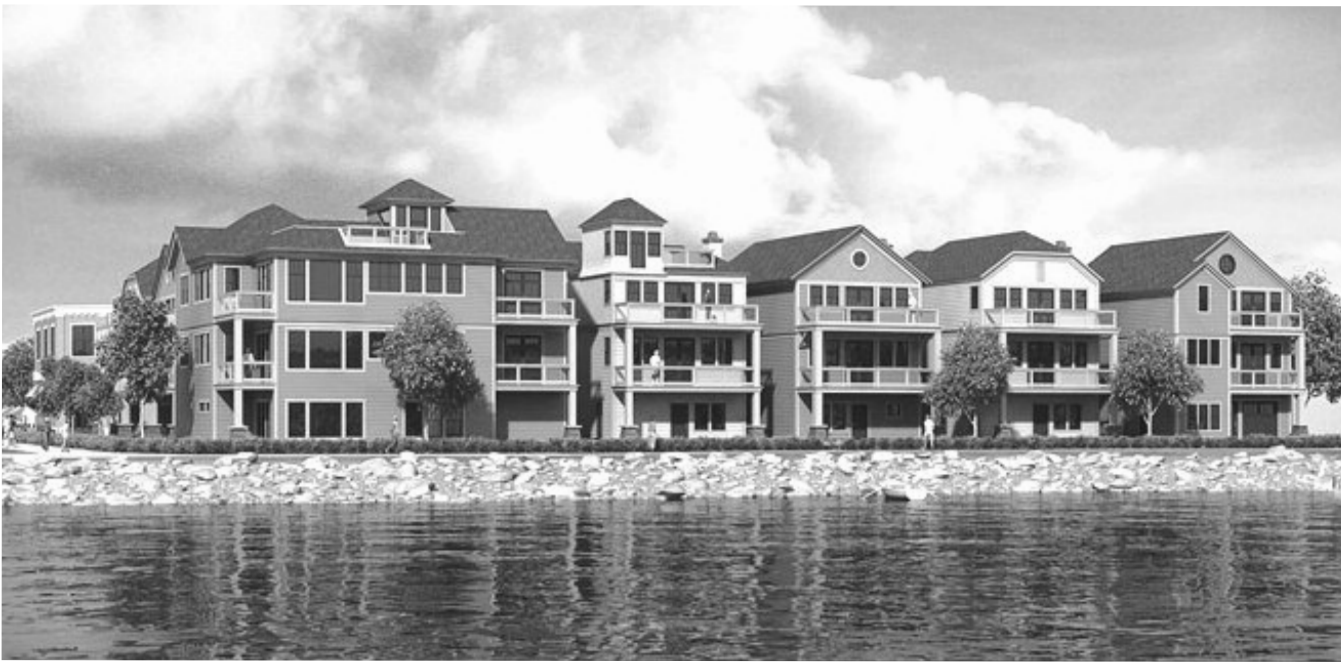
A signing ceremony was held on August 3rd at the City Hall in Boyne City setting the stage for the start of the next phase of the One Water Street development; a residential project consisting of 13 new three-story condo/hotel/cottage buildings containing 15 separate units. Rendering courtesy of Kidd & Leavy Real Estate.
